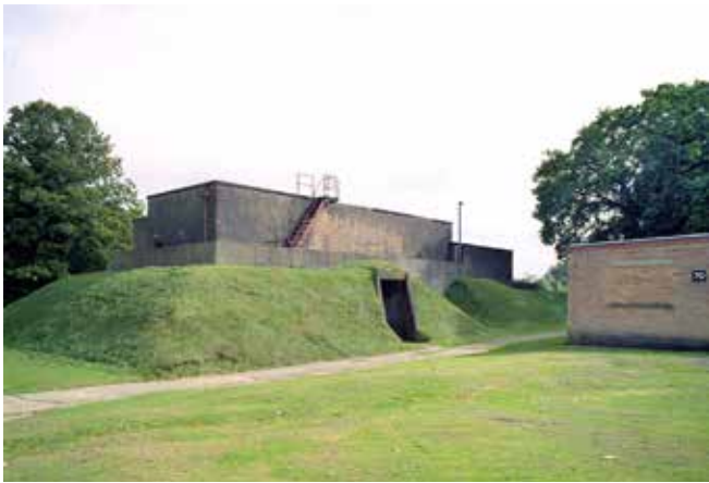
The Sector Operations Centre at Carver Barracks in 2003. Photo Nick Catford
